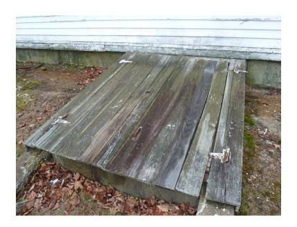
The bulkhead was built with poured concrete and blocks in the 1950's. The current cover is made of tongue and grove boards, in very bad condition and leaking. Modern tongue and groove boards are not expected to last. We propose to use T1-11 exterior plywood with simulated 8" boards, replicating the design used at 4 South Royalston Rd. It will be painted white (as was the existing one) or green (will not show dirt).
