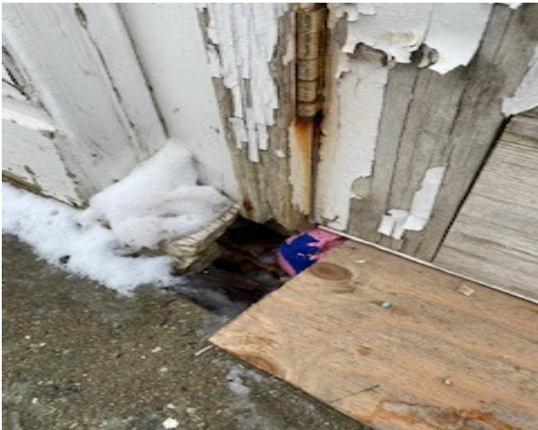
Left side of damaged threshold
