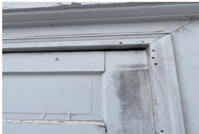
Right side gap between door and frame
