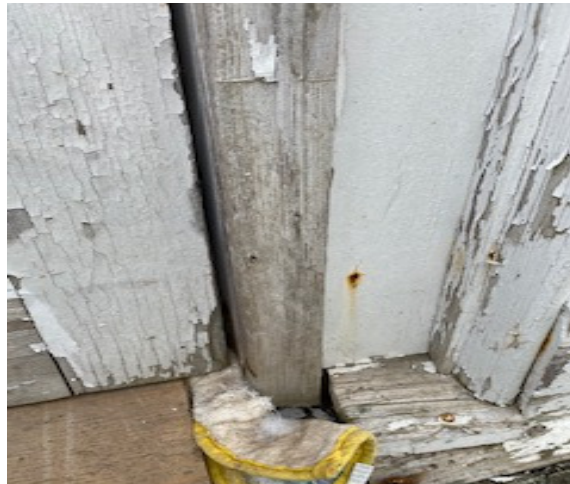
Right side of damaged threshold
