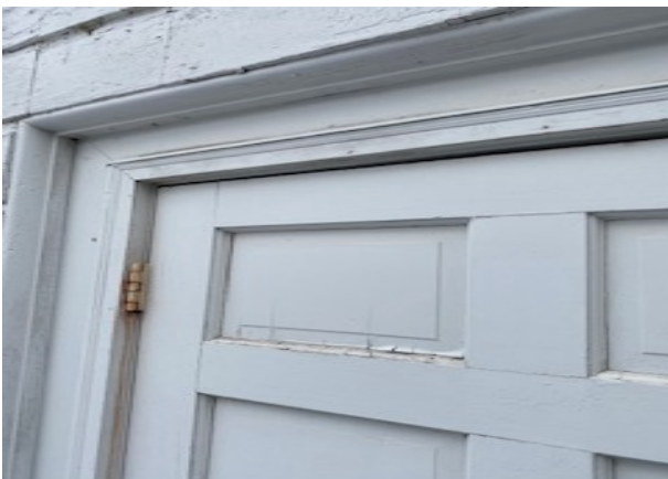
Left side gap between door and frame
